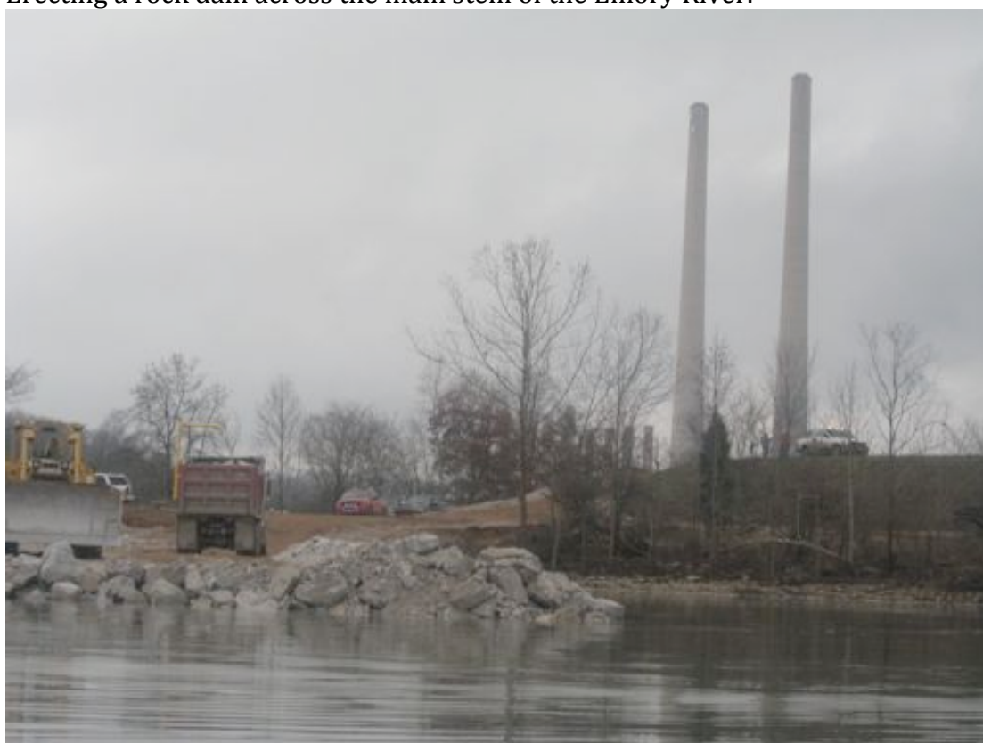
Erecting a rock dam across the main stem of the Emory River.
