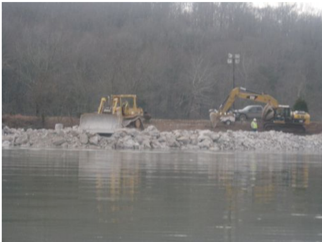
Erecting a rock dam across the main stem of the Emory River.
